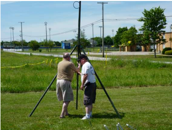
Michael KG4ZPZ and Roman KE6YCW set up the mast and dual-band j-pole antenna used for the packet station.
