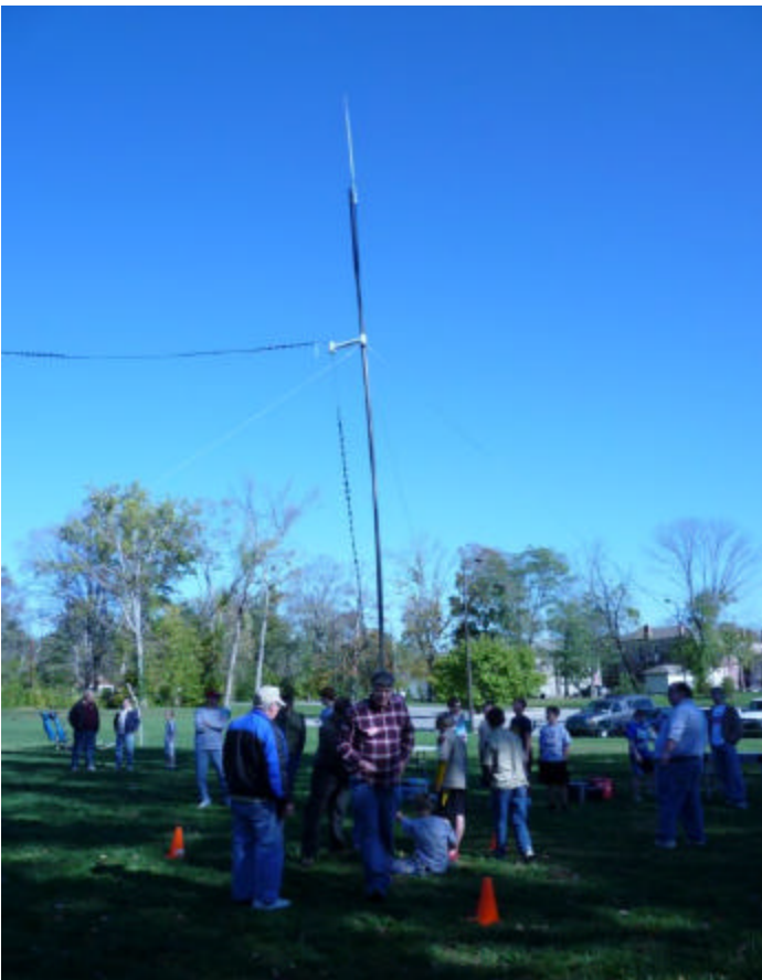
Scouts man both the mast base and assist in the placement of stakes to secure the guy-wires for the main HF mast.
